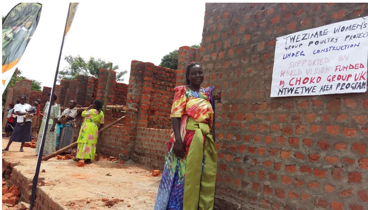
Photo 6: The chairperson of the group stands in front of the building under construction.
